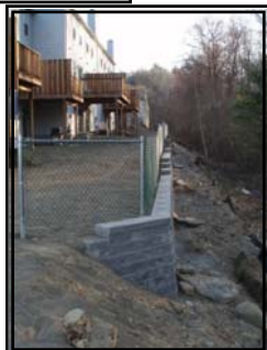
Wall and fence at Bldg. #7
